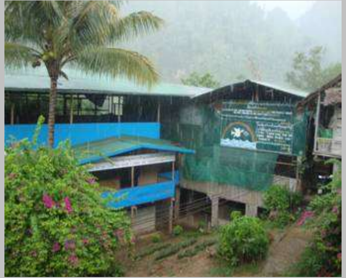
1st & 2nd flrs -classrooms. 3rd flr i-students' dorm & music room. Adjacent building-main hall, , worship
